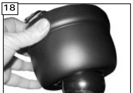
Place canopy over ball and downrod.
